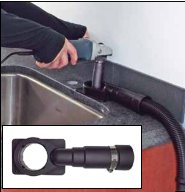
Dust & Water Guard for Core Drilling
