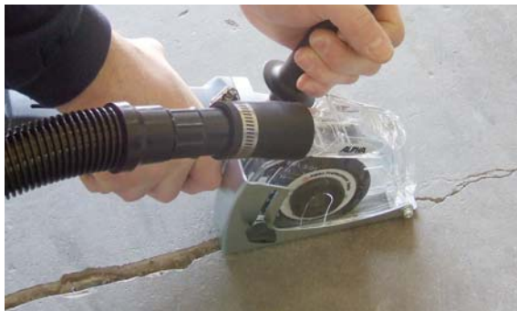
ECOGUARD TYPE W + HOT-ROD BLADE (Crack Chasing)
