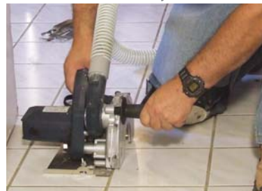
Grout Removal System
