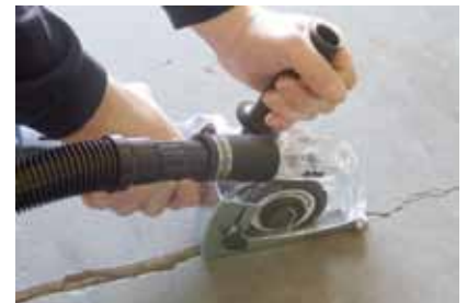
HSG-125 + ECOGUARD TYPE W + CRACK CHASING WHEEL
