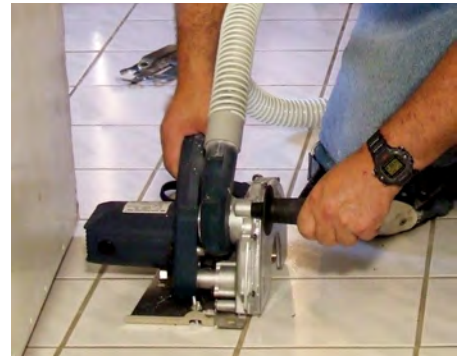
ECOCUTTER (Grout Removal)
