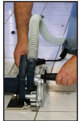
HOT-ROD Removing Grout Lines
