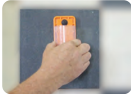
Press the body to the tile and make sure it adheres properly.
