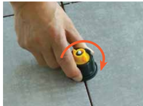
4. Turn Black Base to Tighten
