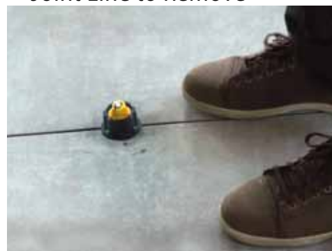
6. Kick the Cap Along the Joint Line to Remove
