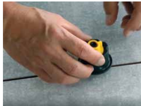
4. Turn Black Base to Tighten
